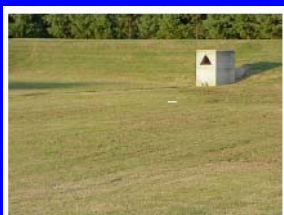
Extended Detention Basin - empty.
